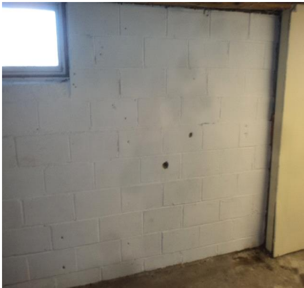
DSC06488.JPG Recently painted foundation wall.
