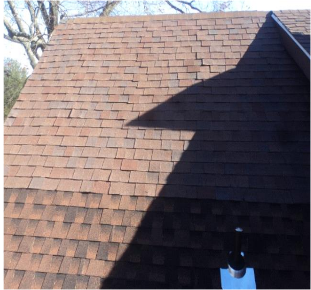
DSC06458.JPG New and old roof covering.
