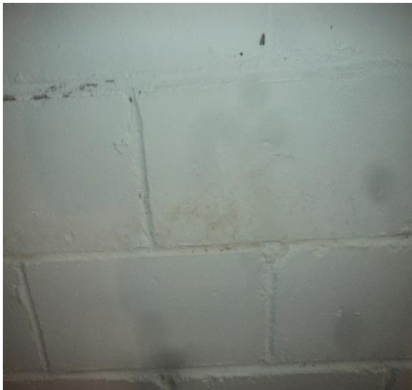
DSC06492.JPG Recently painted foundation wall.
