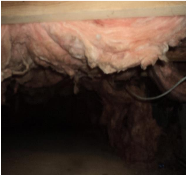
DSC06486.JPG Re-install Insullation in the crawl space.
